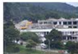
Caption: Vgr4Line (The demolition of the hotel)
