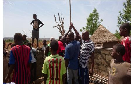
from 4 to 8 pies that we have to lift out of the borehole. Also here, connections are often rusted and worn down, so its sometimes painfully slow. But in the end, we can lift the last pipe with the attached pumping cylinder or motor.
