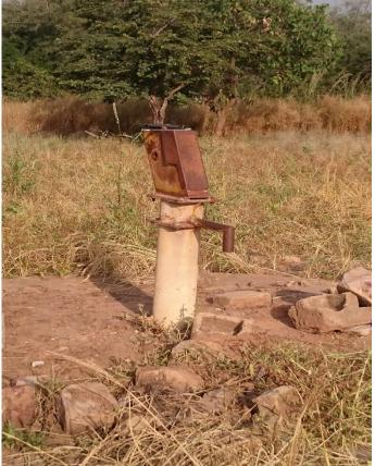
the ground. There is an outer pipe, in which the water is pumped up, and an inner rod, that is connected to the handle on top and the piston down below. This rod makes that, through pumping, the water comes up.
